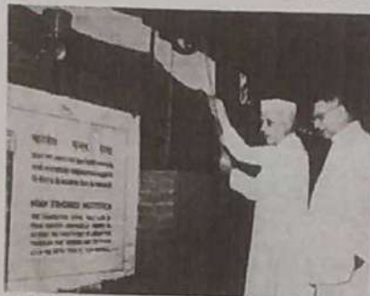
Mr. Nehru laying the foundation stone of the building of the Indian Standards Institute in Delhi on September 22. Mr. V. T. Krishnamachari is also in the picture.
